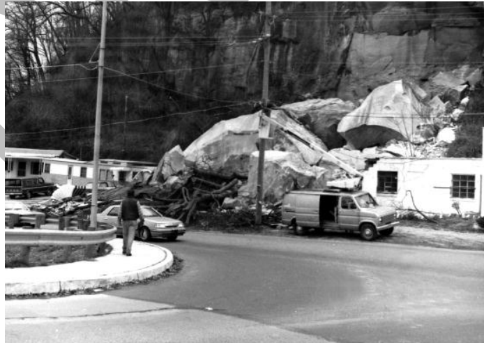
Figure 3: Rock fall in Pomeroy
